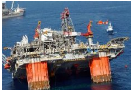
Damage caused by Katrina
